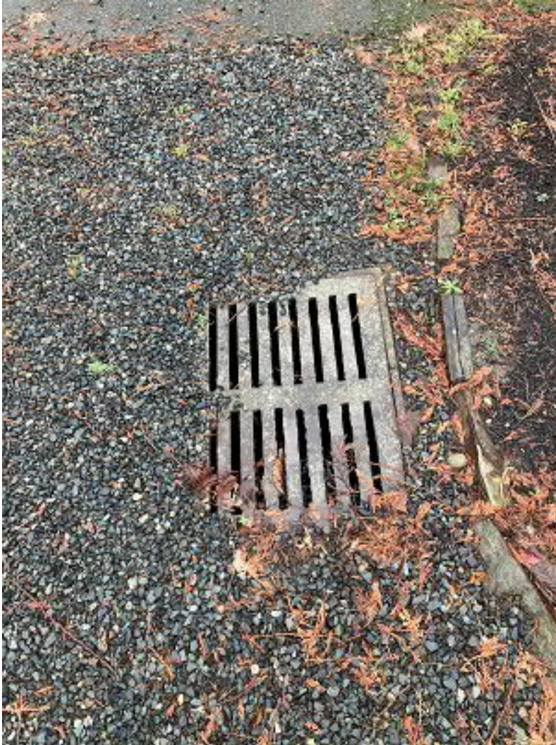
Picture 4: ROW in front of 2416 70 th Avenue SE
