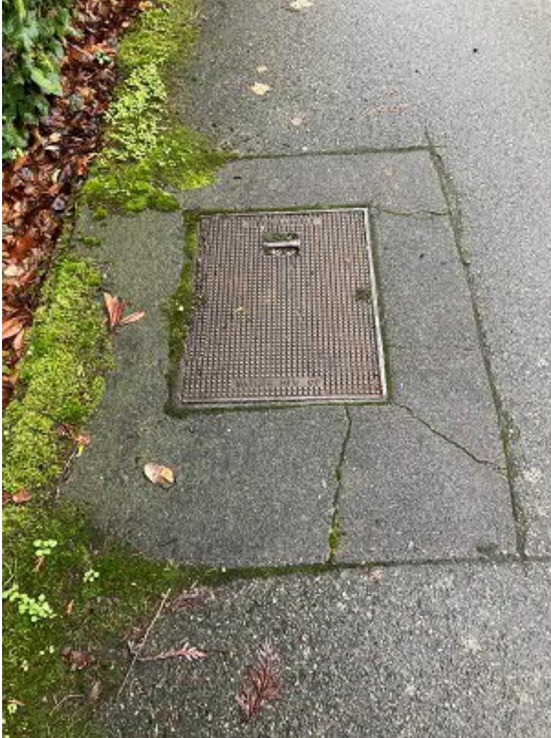
Picture 6: ROW in front of 6605 SE 24 th Street
