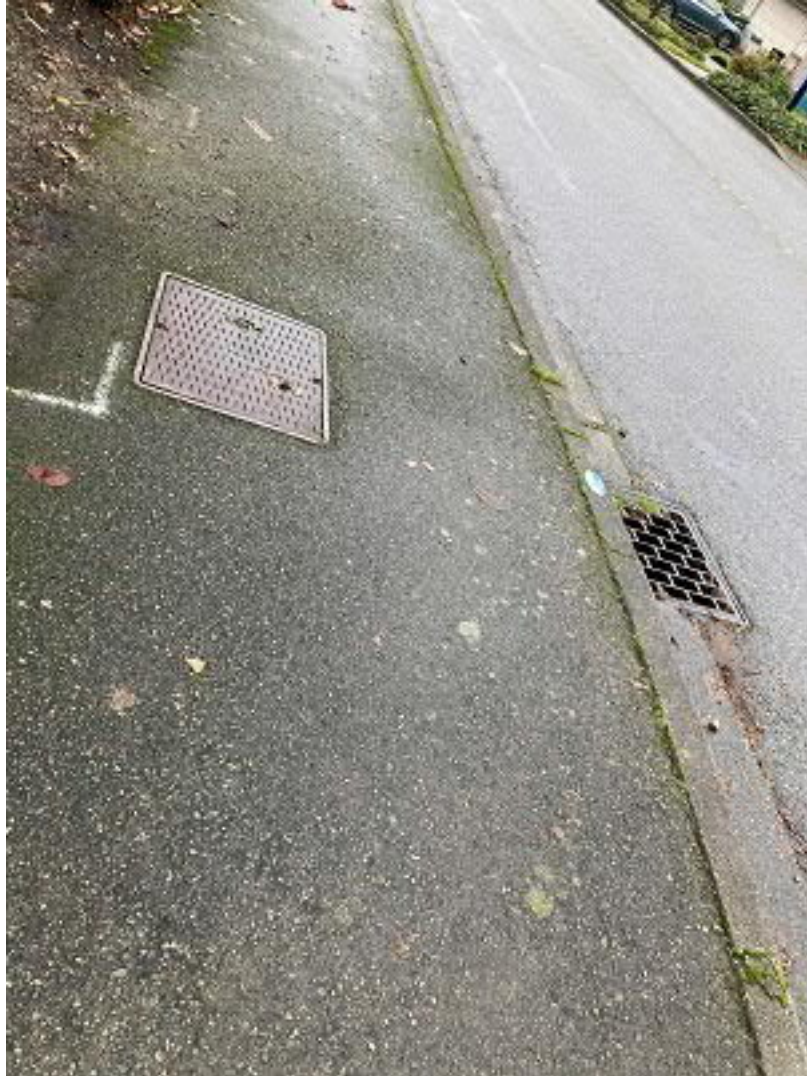
Picture 5: southwest corner of 70 th Avenue SE and SE 24 th Street Existing storm drain has just made a 90-degree turn to the west. The main is under the solid lid.
